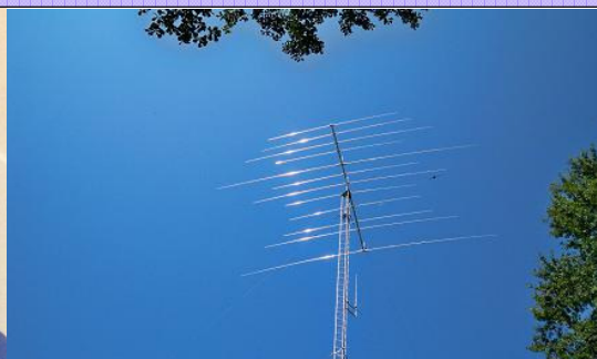
(L) Operating position at K3LB (Center) Chief Op and NFDXA president Larry, K3LB (Right) Optibeam 12-4W at 100 feet; 10M bi-square.
