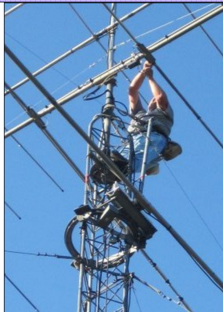
Replacing a broken feed line jumper
