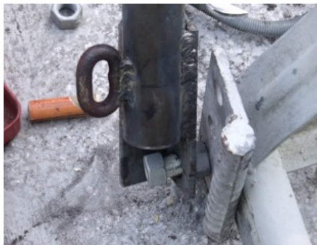
Left—The angle braces being attached by NF4L and K4UTE. Right— Detail of brace bottom. (AB4UF photos)
