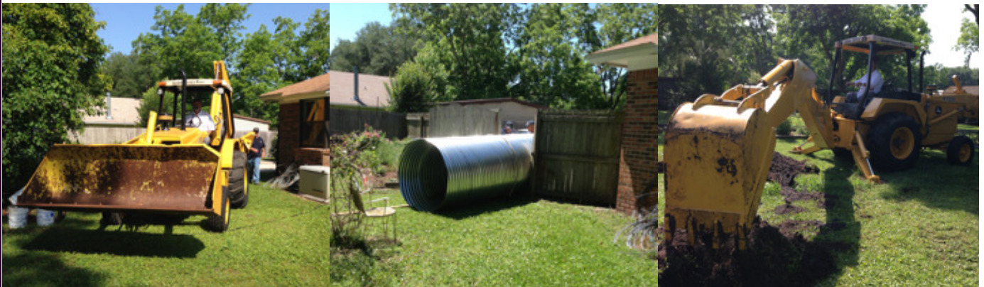
The backhoe squeezes into the yard along with the culvert...and the first bite is taken!
