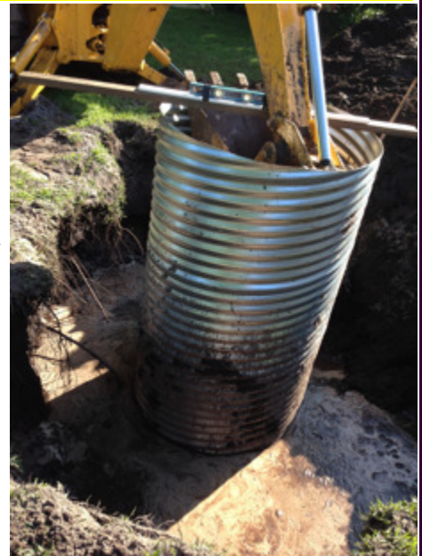
The backhoe squeezes into the yard along with the culvert...and the first bite is taken!
