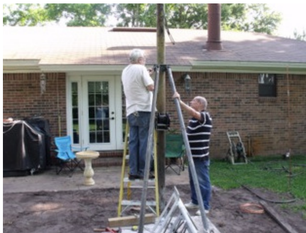
Left—The angle braces being attached by NF4L and K4UTE. Right— Detail of brace bottom. (AB4UF photos)
