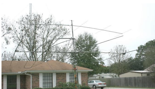
New array set up and waiting for the crane
