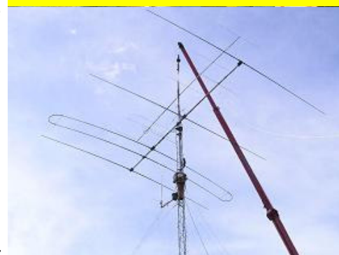
Making final adjustments before releasing the crane attachment
