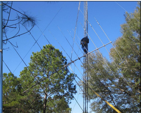
TH-11 being (very) carefully lowered
