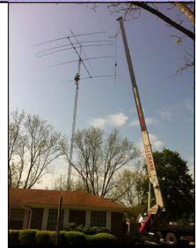
Recent crane repeat 'visit' to NF4L QTH for SteppIR Repairs
